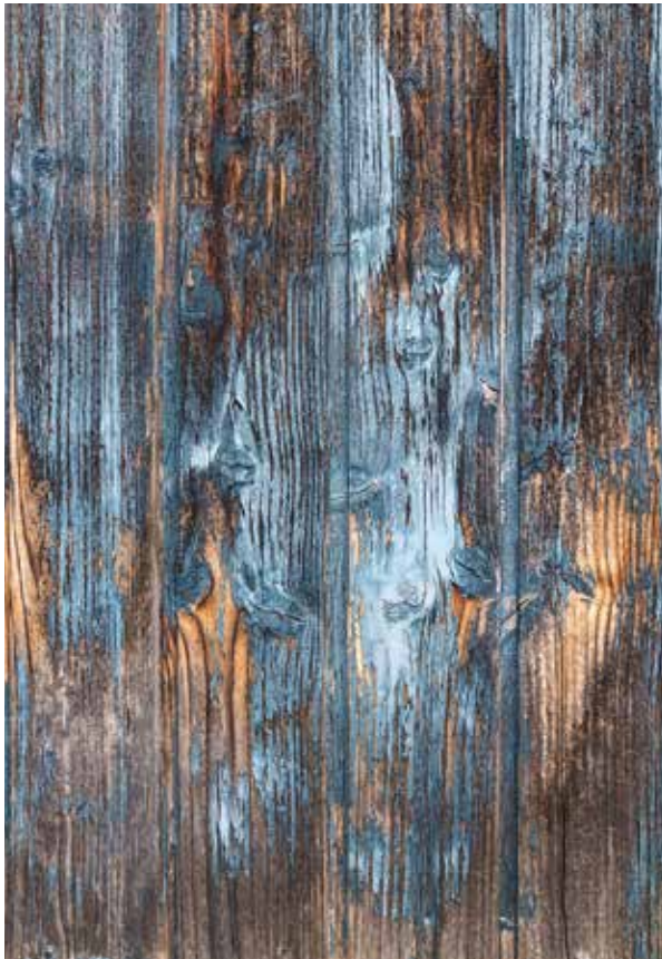
Inevitable side effect: Even with the best protection, wooden façades weather sooner or later. The consequences are sanding and stroking.
